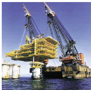
Offshore-Technik Offshore technology Offshore
